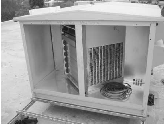
Figure 23.4 Air-to-air heat exchanger (Business Edge)
