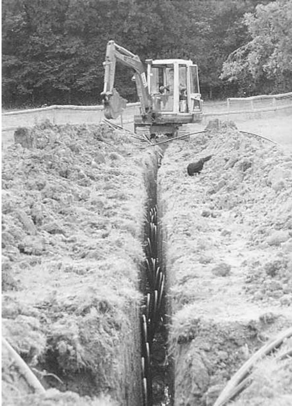
Figure 27.2 Trench for ground source heat pump showing pipe through which glycol solution will be circulated to collect heat (Kensa)
