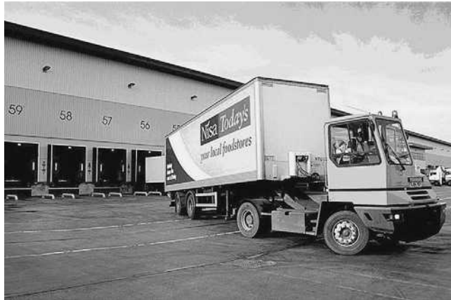
Figure 17.7 Distribution centre (Star Refrigeration)
