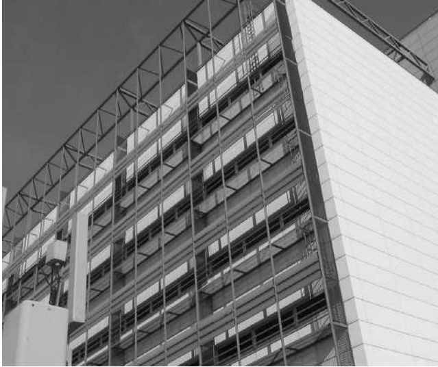
Figure 23.2 Solar shading (Business Edge)
