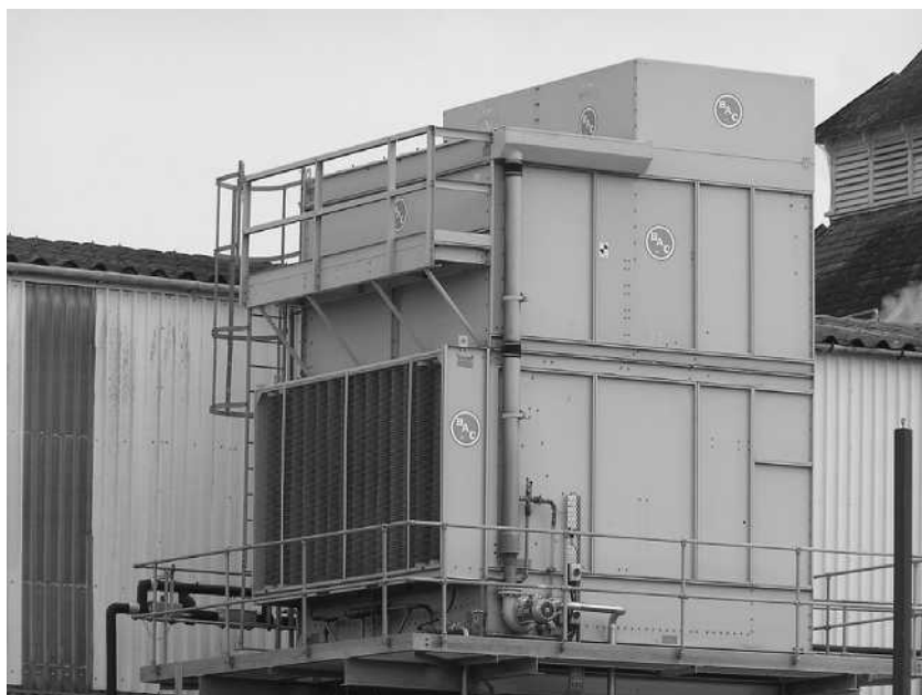
Figure 6.8 Evaporative condenser installation (Baltimore Aircoil)
